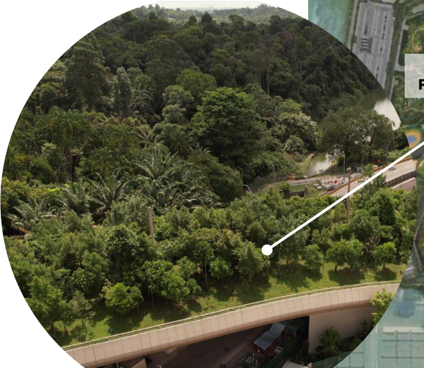
Create new connectivity for native fauna through the Mandai Wildlife Bridge
