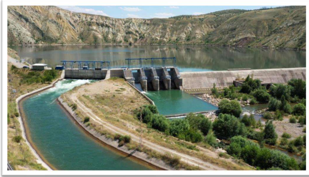
Figure 17. Koyulhisar Hydro Electric Power Plant
